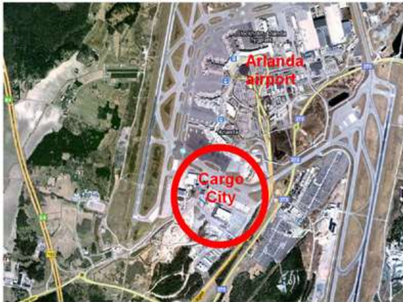
Figure2-2 Aerial view of the Stockholm LTPN
